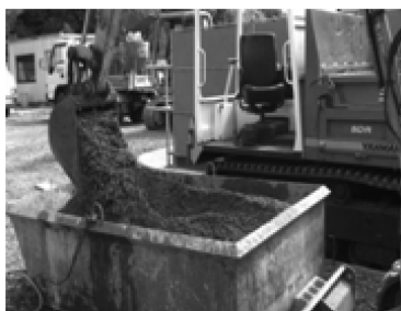
Fig. 2 Mixing of POC in a bucket with backhoe
